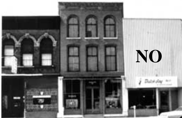
Impact of inappropriate alterations on historic storefronts (the storefront on the right has been totally obscured by a "modern" front added in the 1950s. Photo: NPS files)
